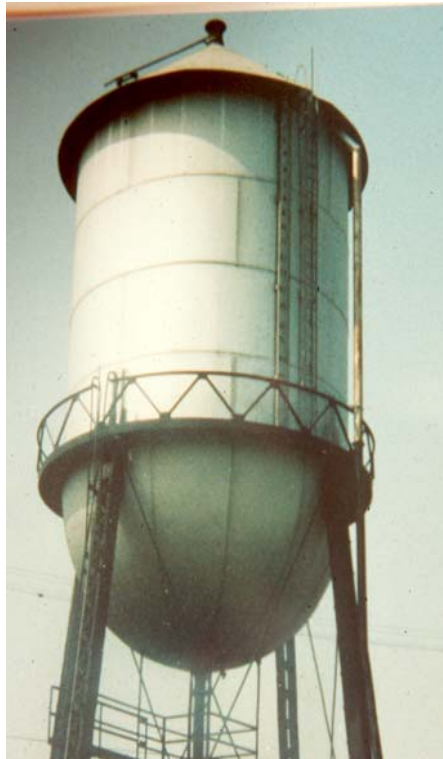
The first steel tanks were constructed from steel or wrought iron plates fastened together with rivets. World War II accelerated the progress of electric arc welding. Welding has proven to be more "maintenance-friendly" than riveted construction.
